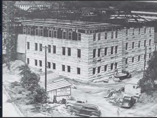
Patton Hall under construction, Fort Riley, Kansas
