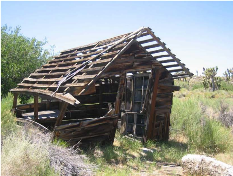
Photo 4. Cabin at China Garden Springs. View to the west.
