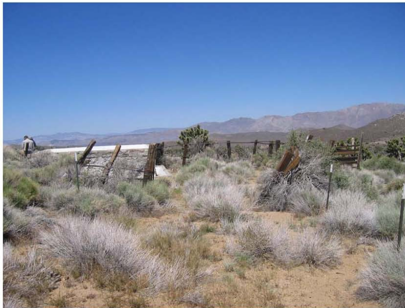
Photo 4. Corral attached to the CCC stock water tank at Cole Spring. View to the NE.
