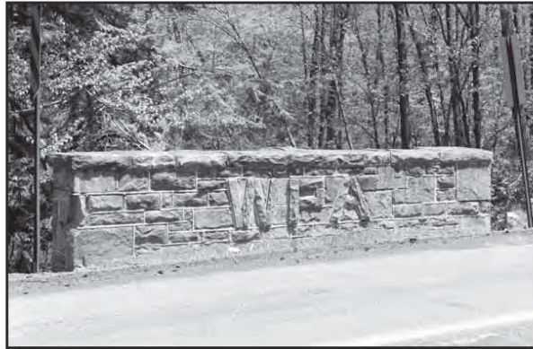
WPA built bridge, Lackawanna County, Pennsylvania
