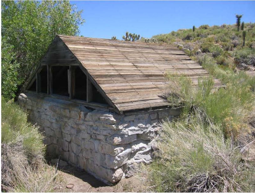
Photo #1. View of CCC stock water tank 2 at Indian Garden Spring. View to the SE.
